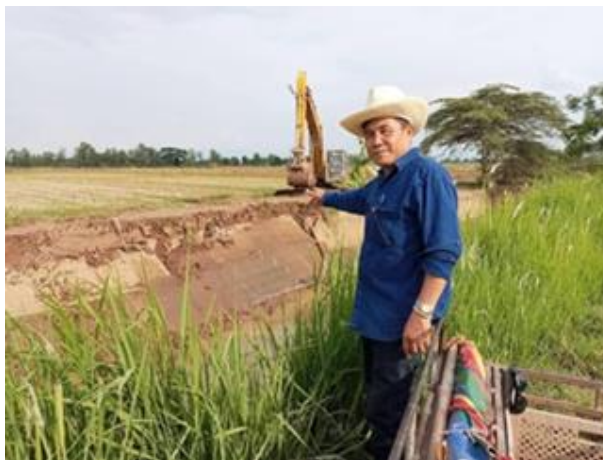
Figure 4. The Head of Hua Mueang Subdistrict Administrative Organization Follows Up on the Canal Dredging Project Implementation
